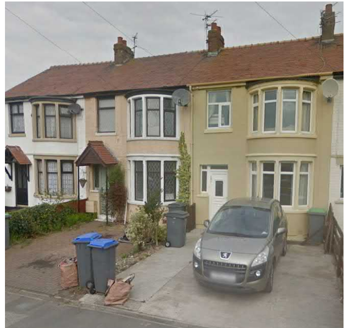
Front boundary/garden removed to provide parking space - School Lane
