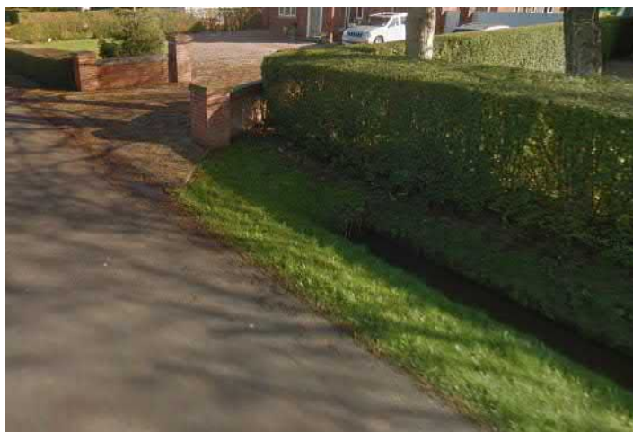
A drainage dyke which has been culverted under a driveway, Division Lane
