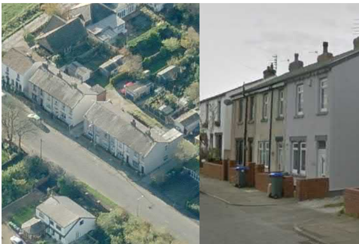
Aerial and photograph of terraced dwellings with short front gardens, Midgeland Rd AECOM
