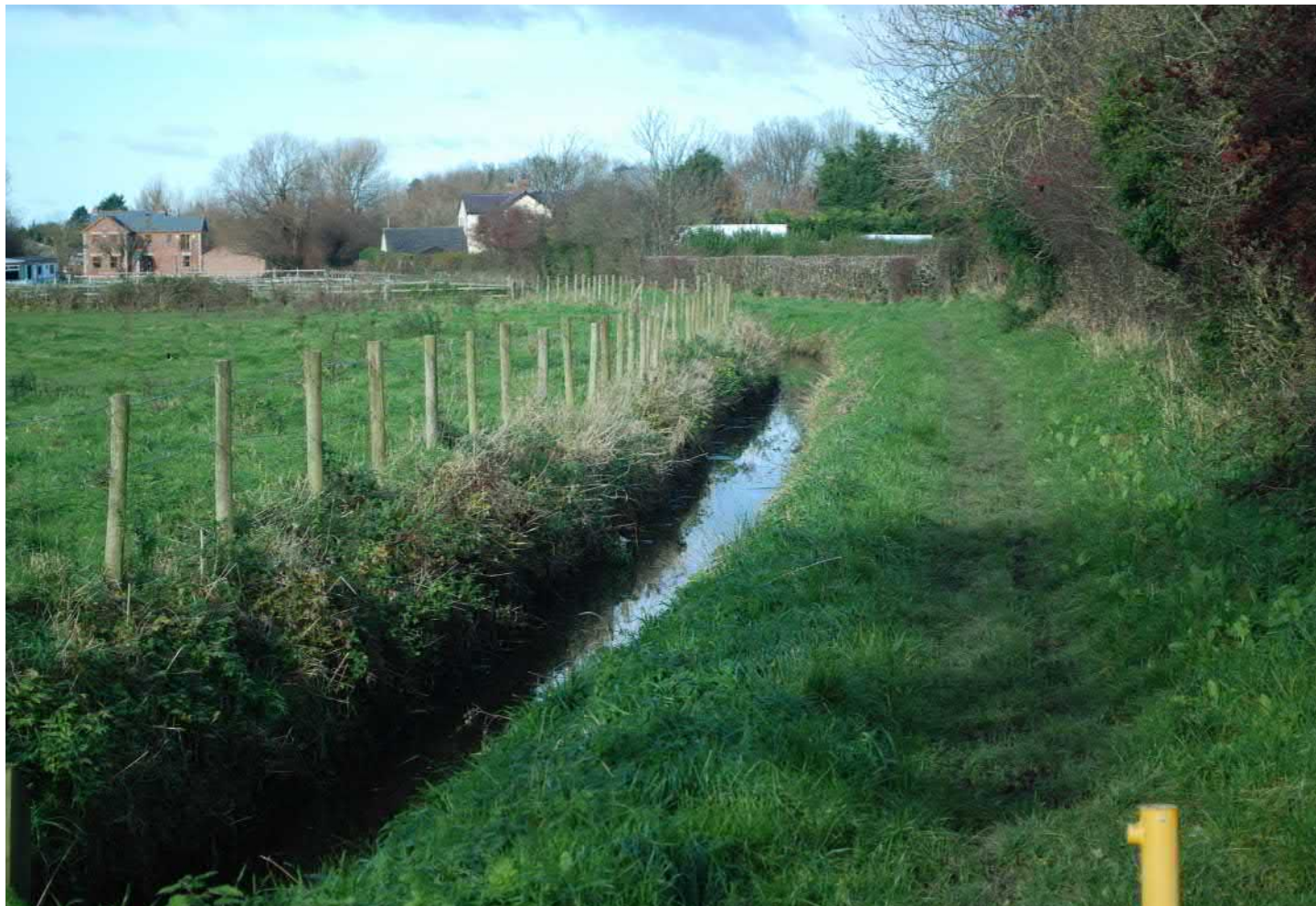
An open drainage dyke alongside the bridleway behind Midgeland Road
