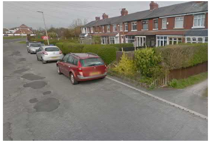
On-street parking, Common Edge Road
