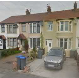
Front boundary/garden removed to provide parking space - School Lane
