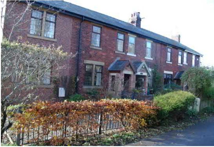
Terrace red brick dwellings, Midgeland Road
