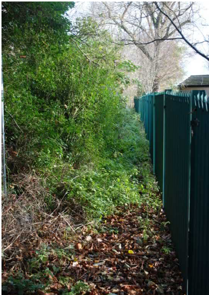
Overgrown public right of way, north of Division Lane
