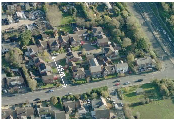
L-shaped, densely enclosed and overcrowded cul-de-sac, Limechase Close, AECOM
