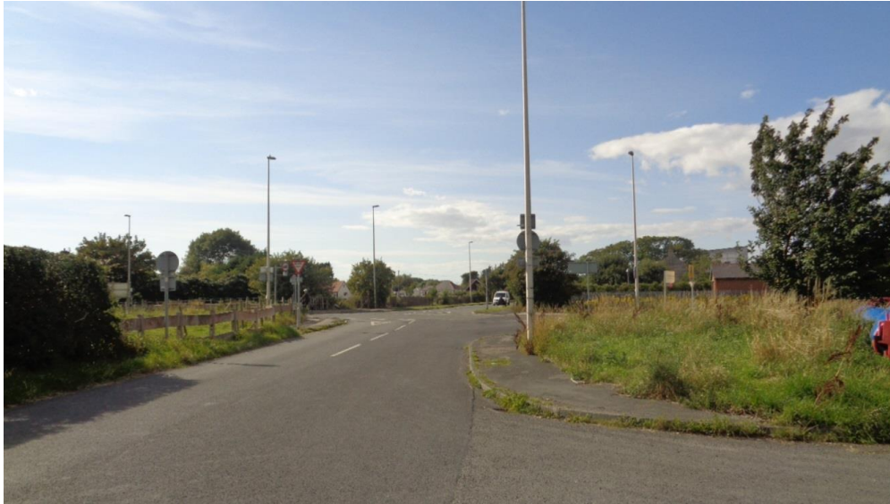
Midgeland Road looking north to the intersection with School Road
