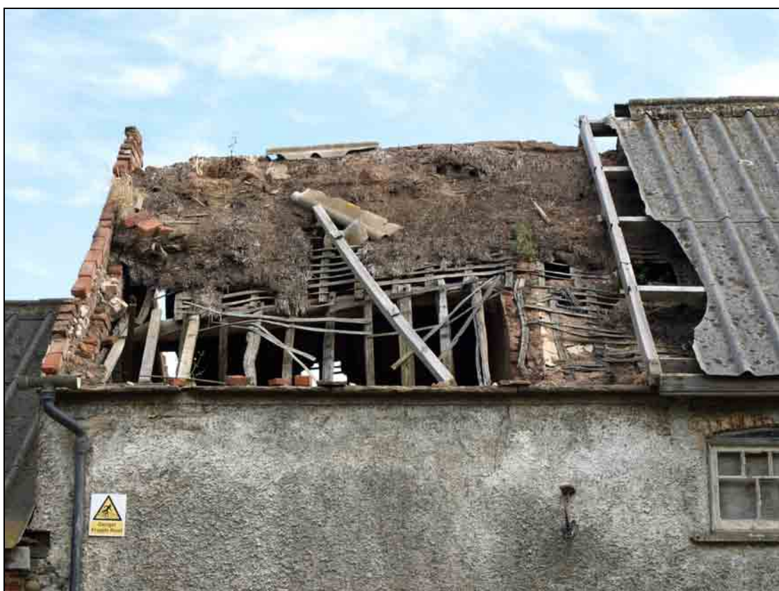
Photo 2: Detail of surviving thatch on Building 1
