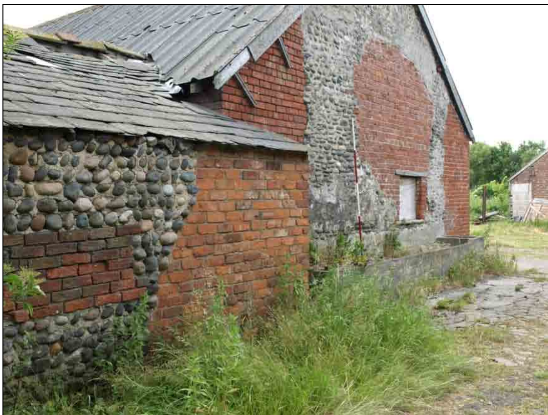
Photo 20: Building 3: shippon, west gable
