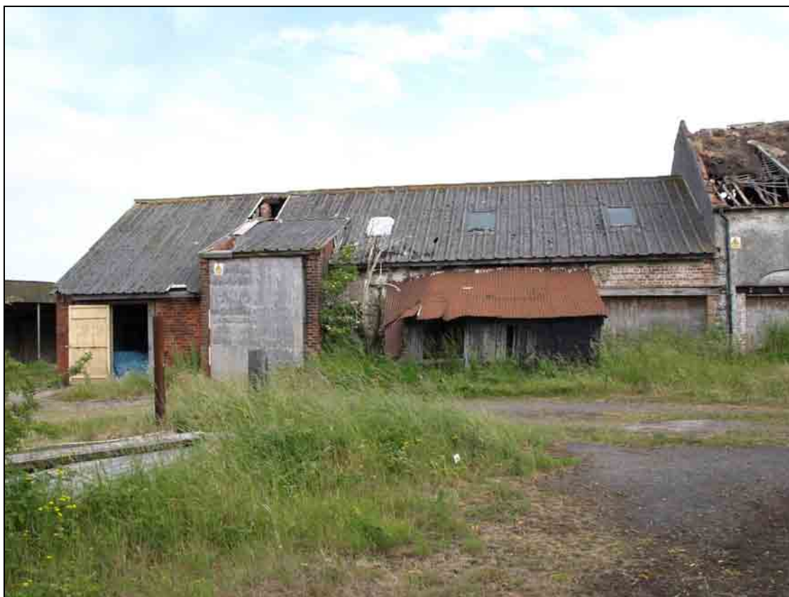
Photo 14: Building 2 and 3: barn and shippon, front elevations
