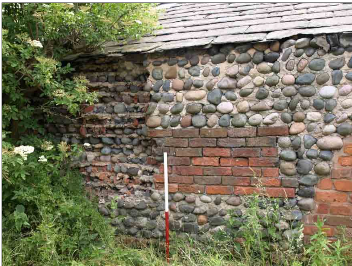
Photo 23: Building 4: detail of brick and cobble west wall
