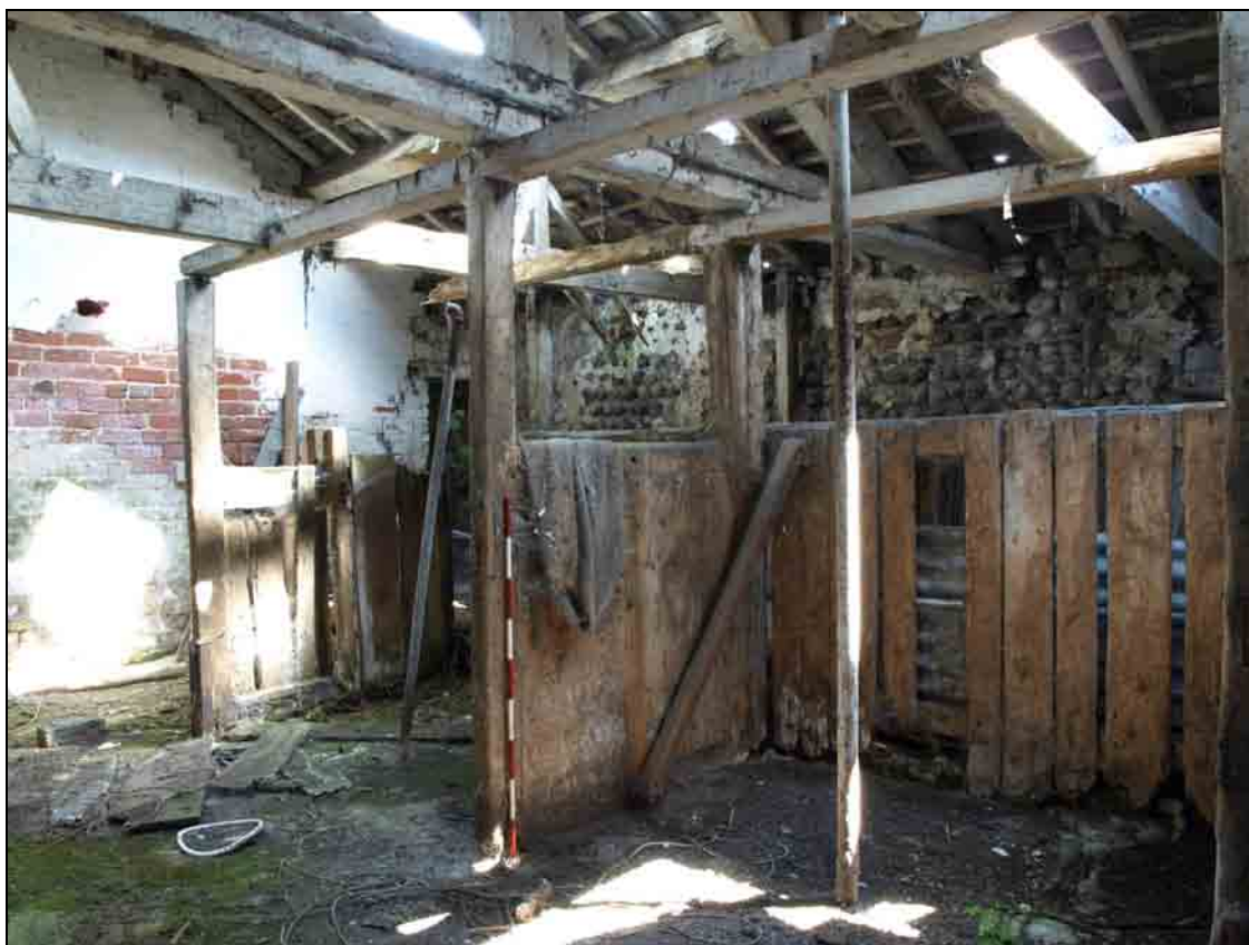
Photo 24: Building 4: interior of shippon, from the south-west
