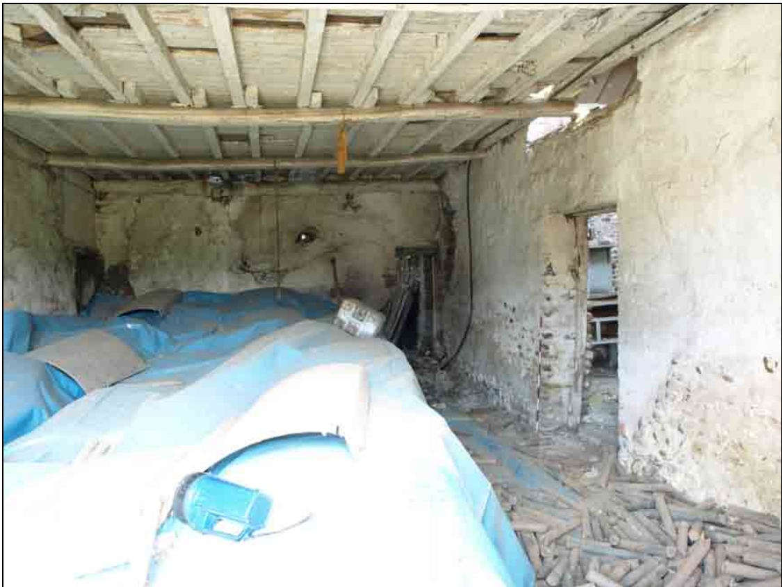
Photo 21: Building 3: shippon interior, from the south
