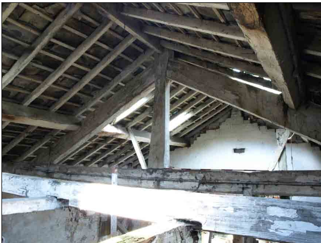
Photo 25: Building 4: roof truss in shippon, from the south-east
