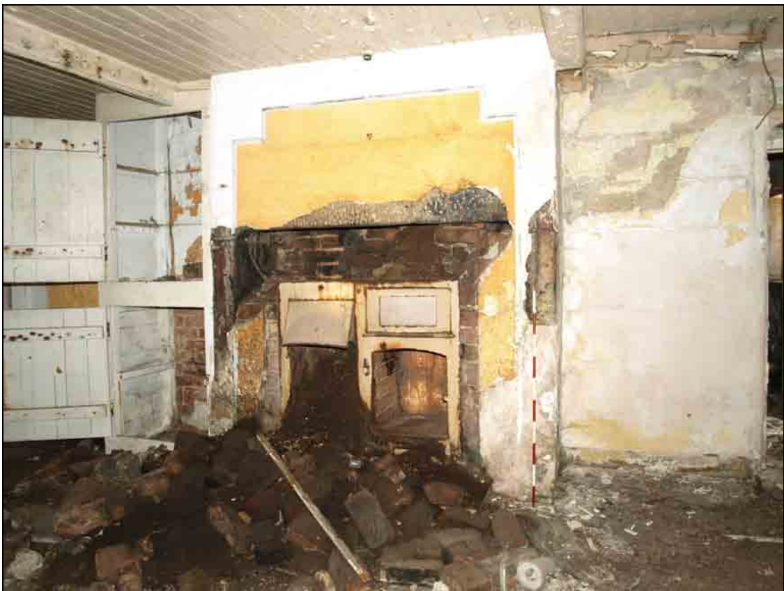
Photo 8: Building 1: kitchen in west part of house (from the west)
