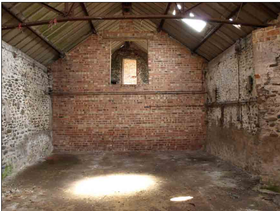
Photo 19: Building 2: interior of barn, from the west, showing modern dividing wall
