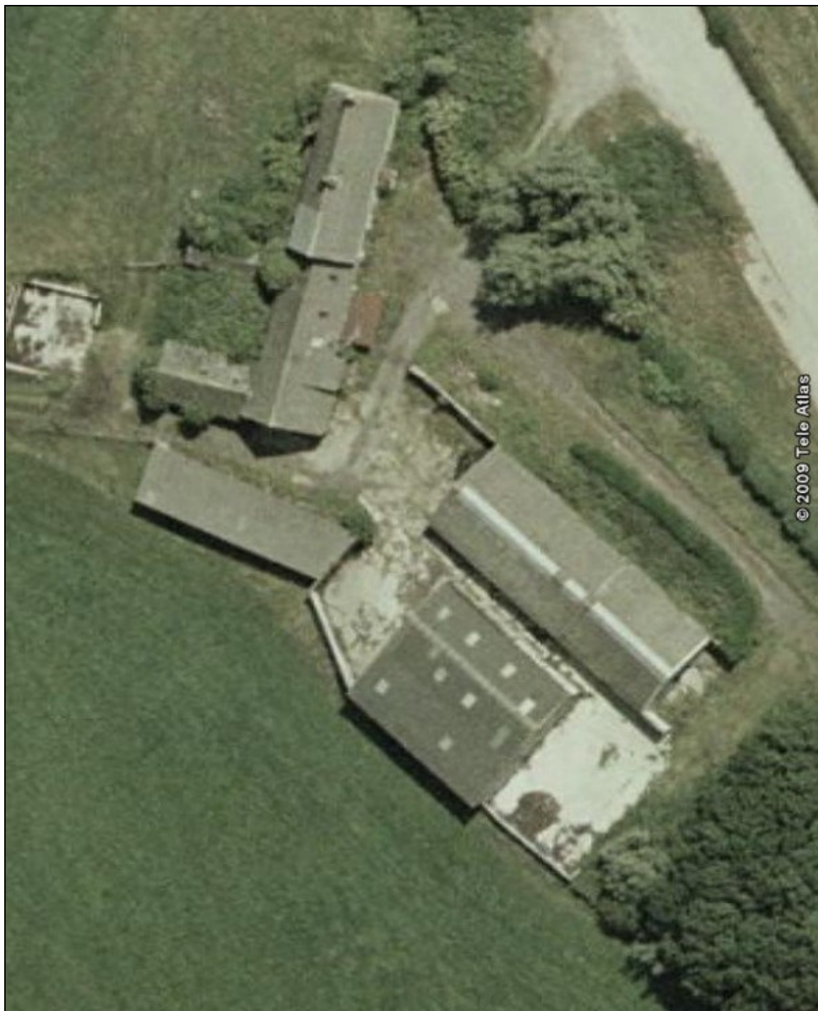
Figure 10: Satellite photograph, early 21st century (Source: Google Earth)
