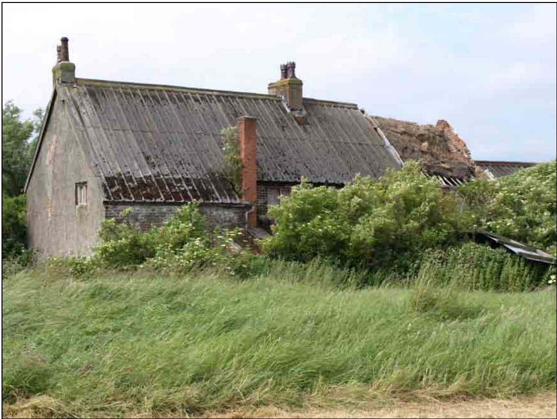
Photo 5: Building 1: house, rear elevation
