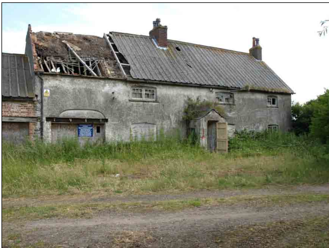
Photo 1: Buildings 1 and 1a: house and former stable, front elevation
