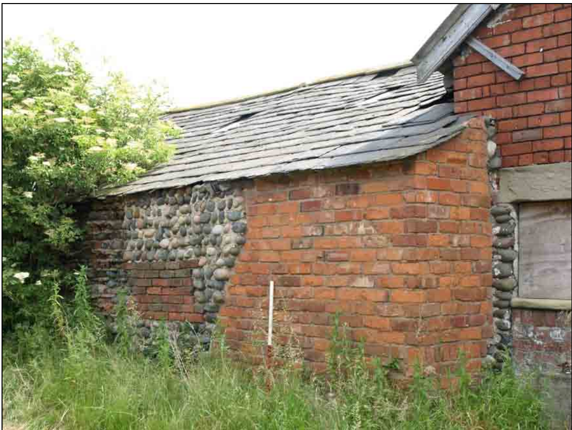
Photo 22: Building 4: shippon, west elevation
