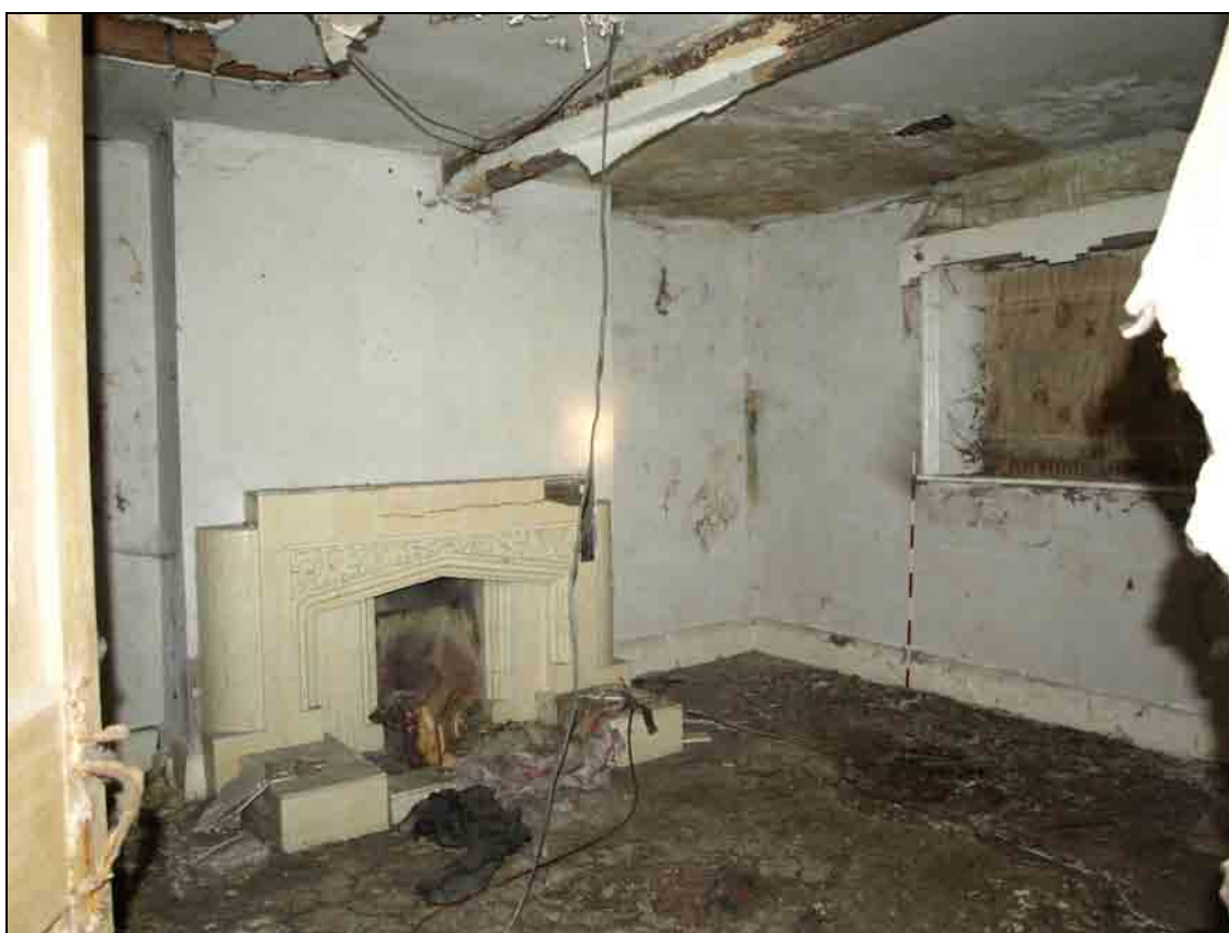
Photo 10: Building 1: parlour in east part of house (from the west)
