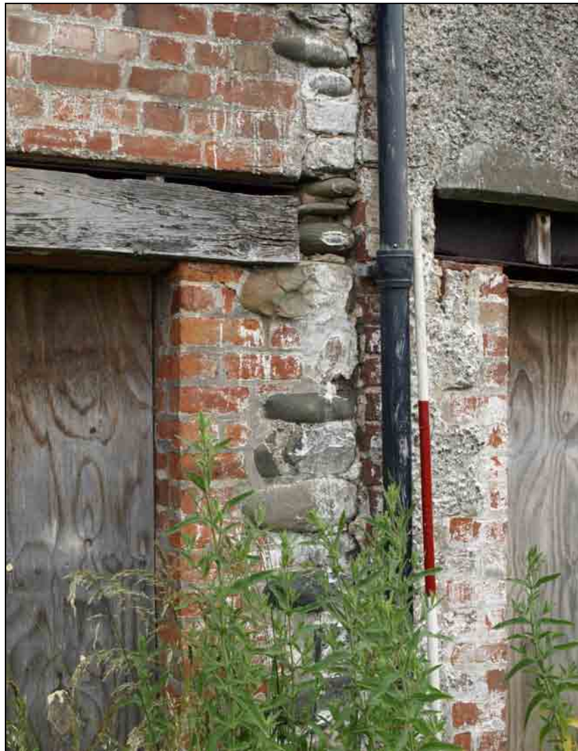
Photo 15: Building 2: detail of butt joint between barn and house
