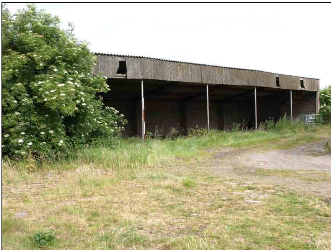
Photo 27: Building 6: modern implement shed, from the east
