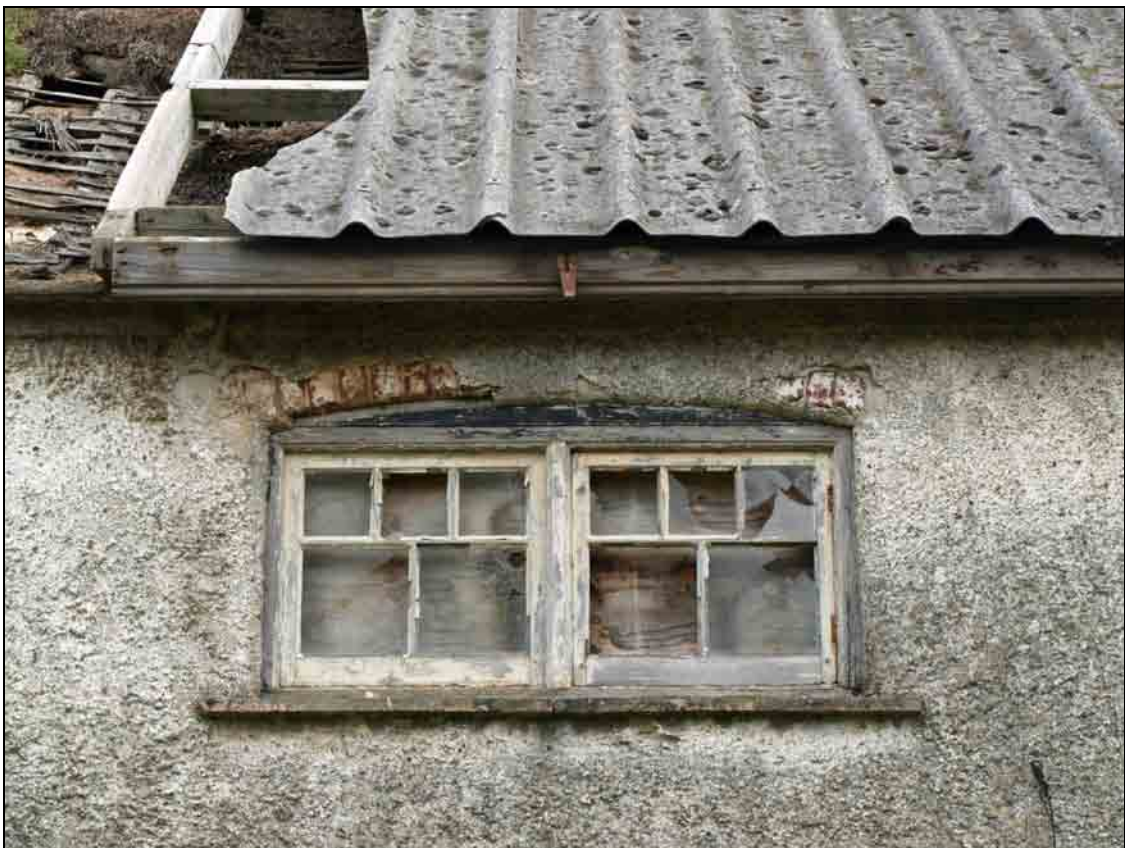
Photo 6: Building 1: typical window in front elevation
