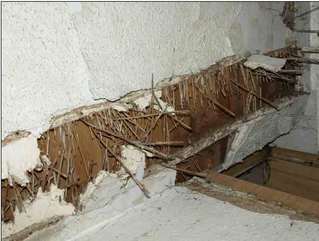
Photo 12: Building 1: detail of plaster and straw ceiling over housebody
