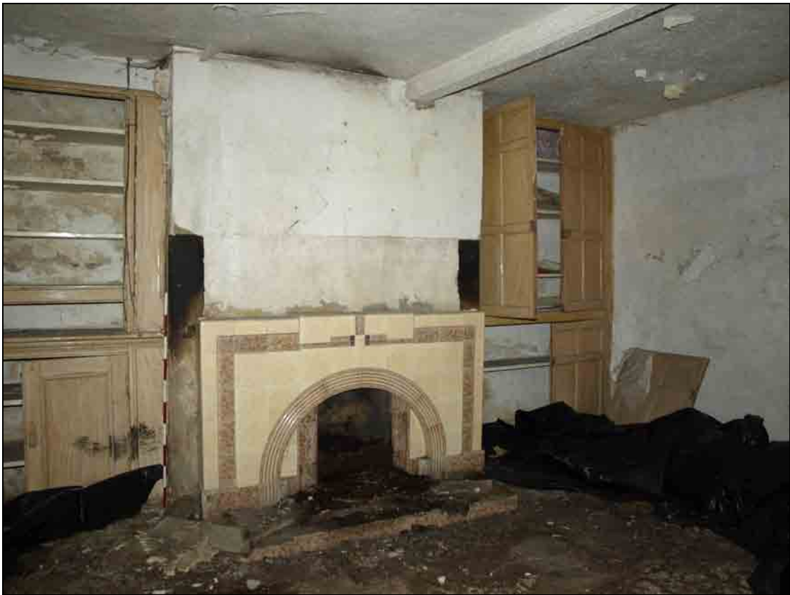
Photo 7: Building 1: housebody in central part of house (from the south-east)
