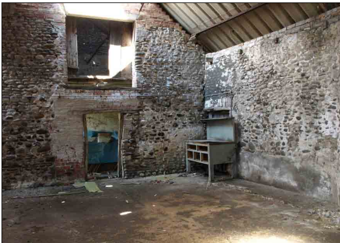
Photo 16: Building 2: interior of barn, from the north-east
