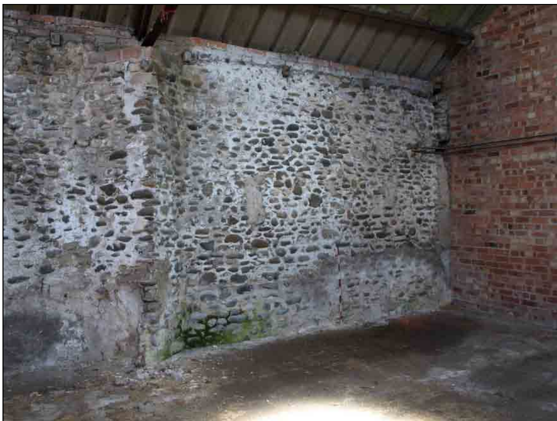
Photo 18: Building 2: interior of barn, from the south-west
